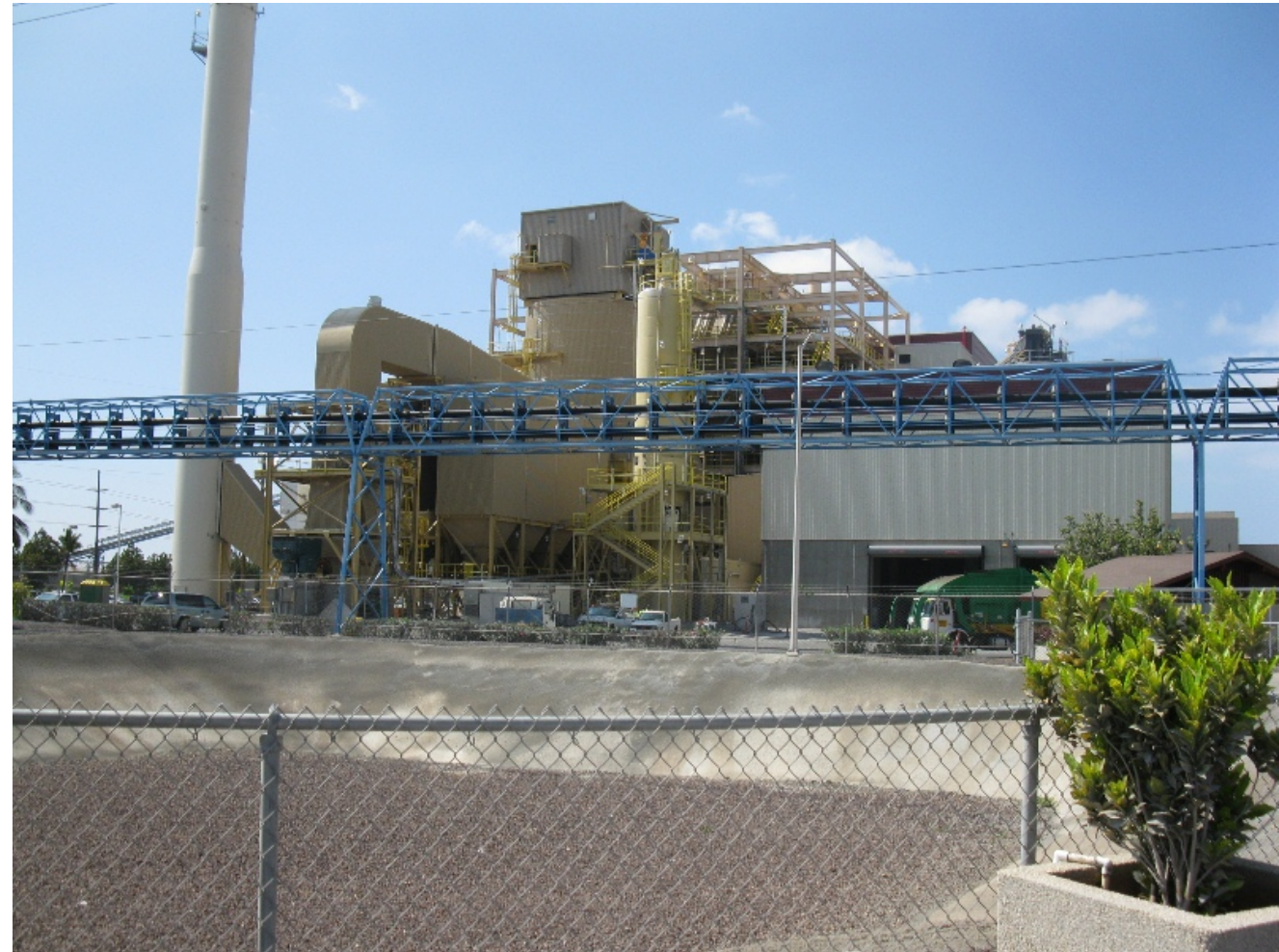
H-Power Garbage to Energy Power Plant
